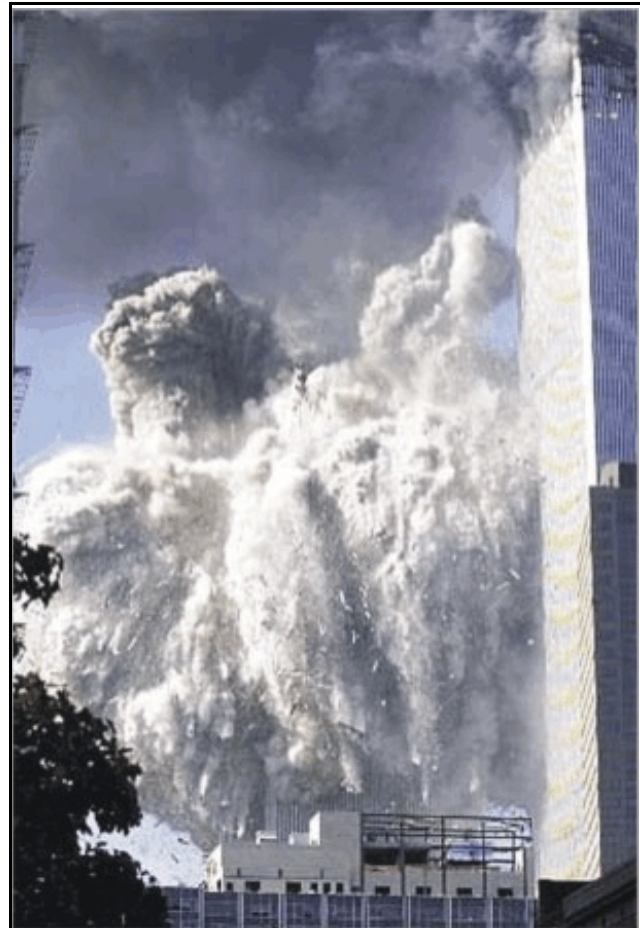
Figure 1 Collapse of the Twin Towers on Sep. 11, 2001 as a tipping point was reached. (Source: University of Sydney http://www.civil.usyd.edu.au/wtc.shtml )
