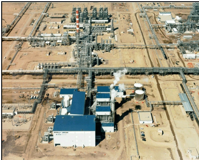
Figure 3 The Joffre Cogeneration facility is the largest cogeneration power plant in Canada. Located east of Red Deer, Alberta, in Western Canada, the power station produces steam, heat and electricity for the NOVA Chemicals petrochemical facility. The surplus electricity of 290 megawatts is sold to the grid. (Source: NOVA.)
