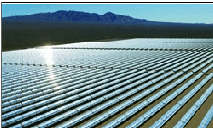
Figure 15 Nevada Solar One started operating in June, 2007, the largest such plant to be built in 17 years. Much smaller than Luz, it generates about 64 megawatts, or enough power for about 14,000 homes. (Source: ACCONIA)
