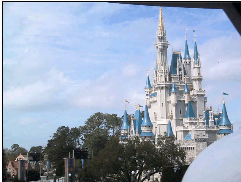
Figure 2 At Walt Disney World, waste heat from electricity generation is used to provide air conditioning.
