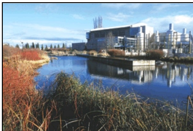
Figure 12 The Portland, Oregon, Columbia Boulevard sewage plant makes methane, or natural gas, from human waste. It is fed in to a fuel cell, a device that generates chemically, making enough electricity for about 40 homes, saving the city about $60,000 a year. (Source: Oregon Chapter, American Society of Landscape Architects)
