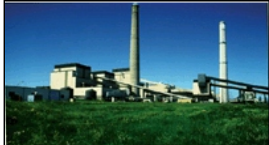
Figure 3 America's second-dirtiest power plant in terms of carbon dioxide, Sherco in Minnesota. Owned by Xcel, it emits 2,797 pounds of \text{CO}_2 for every megawatt hour generated and dates to 1976–77.
