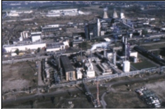
Figure 7 The Schwarze Pumpe IGCC plant in Spreewitz, Germany, gasifies a variety of wastes, ranging from scrap plastic to junked railroad ties, to produce electricity, steam, and chemical feedstock.
