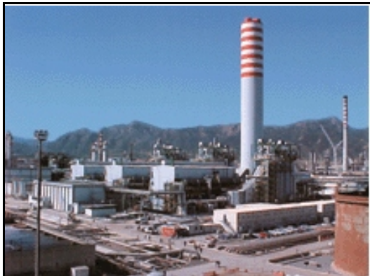
Figure 6 The IGCC plant at the Saras Oil Refinery in Sarroch, Italy is the second largest European refinery. It makes 551 megawatts of electricity, enough for about 120,000 U.S. homes, as well as 285 metric tons of process steam for the refinery, as well as 20 million standard cubic feet a day of hydrogen feedstock.
