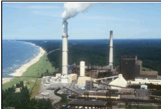
Figure 4 America's dirtiest power plant in terms of oxides of nitrogen. Baily, owned by Northern Indiana Public Service and built in 1962, emits 9.66 pounds of \text{NO}_x for every megawatt generated.
