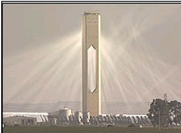
Figure 14 Located in Seville, Spain, this 40-story "power tower" will eventually provide electricity for the city's 600,000 residents, producing no air pollution whatsoever. (Source: BBC)
