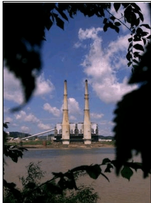
Figure 5 America's dirtiest power plant in terms of sulfur dioxide. Gallagher, owned by Public Service of Indiana and built in 1961, emits 40 pounds of \text{SO}_2 for every megawatt hour of electricity generated.
