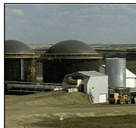
Figure 11 A power plant in Alberta, Canada harnesses the power of solid cow manure. The $8-million system starts with manure, adds water and heat, and then lets the mixture stew without oxygen, producing methane, or natural gas, that is burned to generate electricity. (Source: Canadian Broadcasting Corporation)
