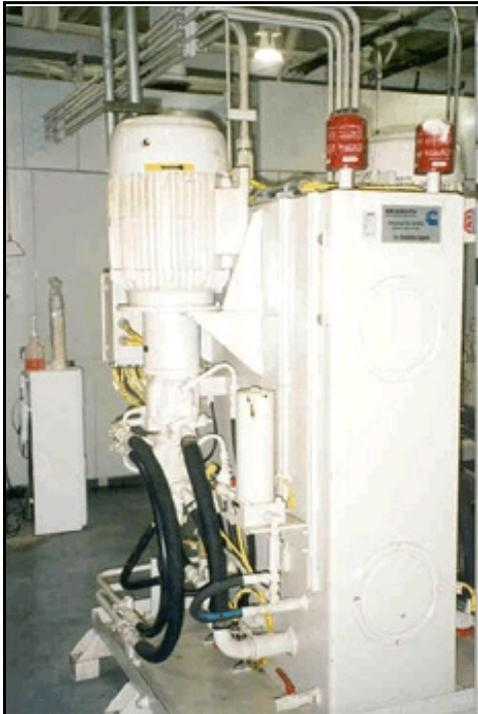
**Figure 5** Engine manufacturer Cummins replaced 296 motors ranging from 1 to 125 hp with premium-efficiency versions at its Midrange Engine Plant in Walesboro, Indiana. Although the new motors were only a few percent more efficient than the standard motors they replaced, they reduced power costs by \$80,000 per year.
